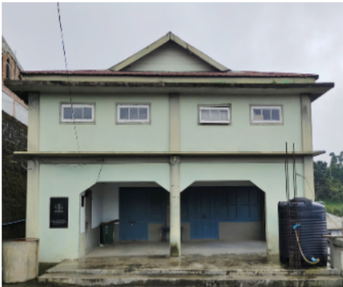
Polling Station Building Front View
